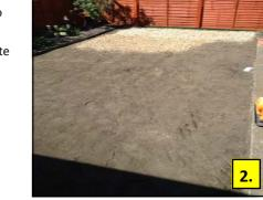
aggregate to a depth of around 25mm, or until flush with the top of the timber frame. Level the area again using a compactor plate / roller or wood batten.
