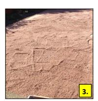
Create a base using Type 1 hard-core, to aid with drainage ,to a depth of around 50mm. Compact using a compactor plate or roller.
