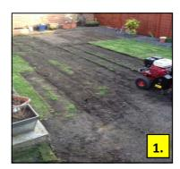
Remove your existing turf to a depth of approximately 75mm. If a frame is required, treated wood timber battens can be installed around the perimeter.
