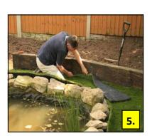
the grass pile on each roll is pointing in the same direction. Butt any edges together and weigh down to avoid movement. A Stanley knife can be used to easily cut and shape the grass as required.
